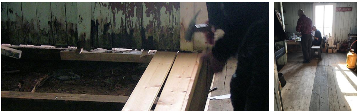
Left: The floor continues under the wall. Right: Finished floor.
