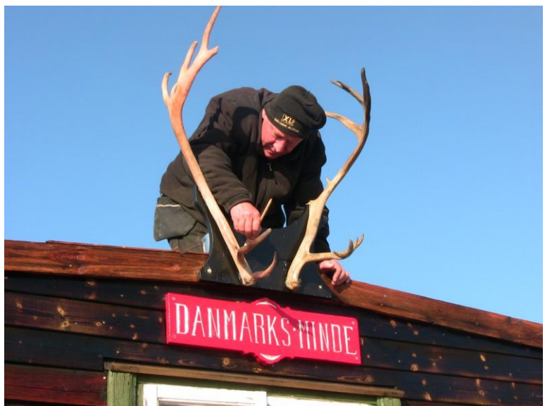
The antlers are repaired and mounted.
