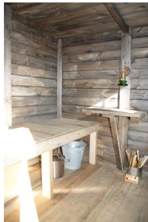
Restoration of Blæsenborg [443]. The old floor was rotten and had to be replaced. A new bunk and table similar to the previous were made for the inside.
