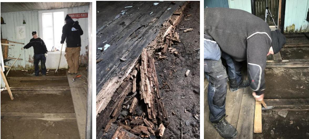
The joists are exposed, where the floor has been broken up. Many boards disintegrate.
