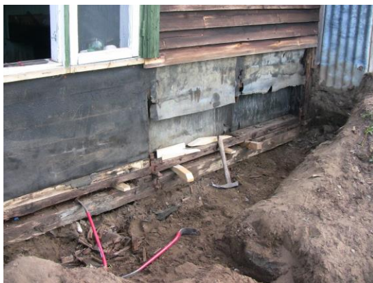
Left and middle: The rotten posts below the window. Right: The new wood is scorched with a gas burner to give it an authentic appearance.
