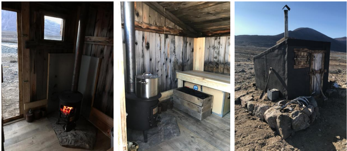
Antonsens hytte [444] after restoration. The old stove was located on a flat rock of ½ m 2 , and the floor consisted of earth and rock. We chose to put a wooden floor, and the flat rock was reused for the new stove.
