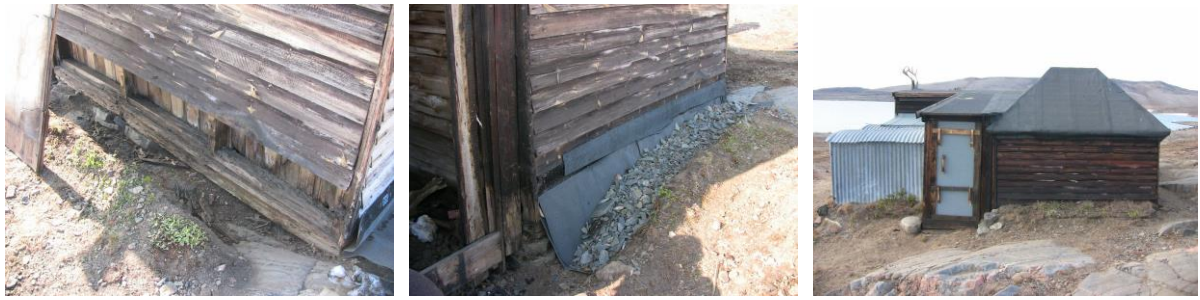
Left and middle: East wall before and after restoration. Right: Finished wall with backdoor.
