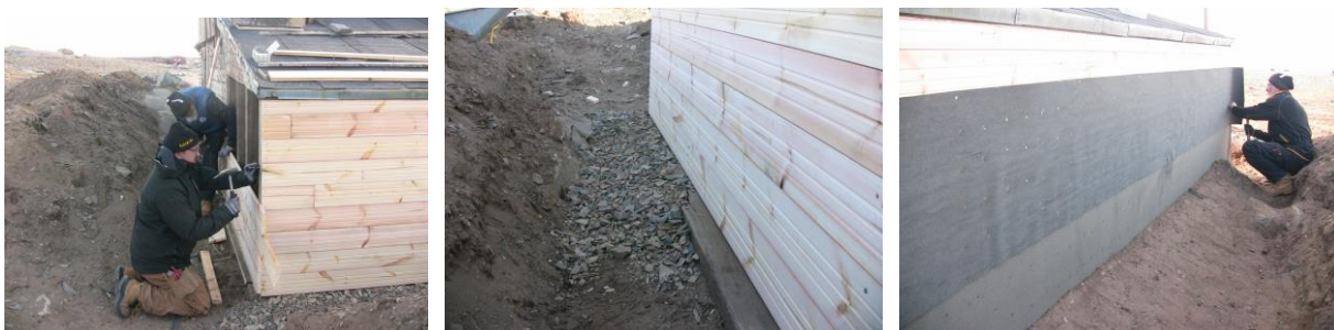
The new wall with floorboards, drain made with chippings and roofing felt.
