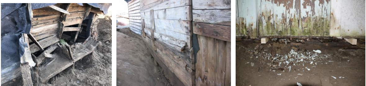
There were rot and decay in the lower areas of the walls.
