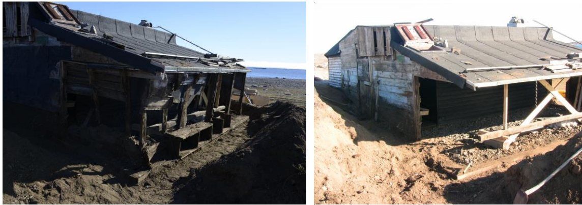
Left: The boxes in the bank. Right: Roof is supported
