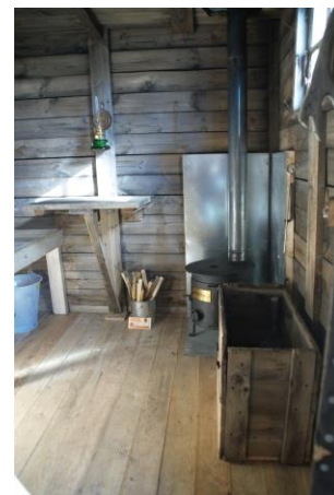
Restoration of Blæsenborg [443]. The old floor was rotten and had to be replaced. A new bunk and table similar to the previous were made for the inside.
