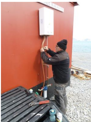
Left: Installation of water heater for Tolvmandsbarakken. Middle: Fitting of refrigerator and stove. Right: Running hot and cold water makes kitchen work much easier.
