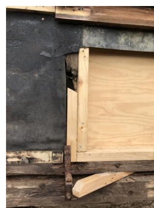
Left and middle: The rotten posts below the window. Right: The new wood is scorched with a gas burner to give it an authentic appearance.
