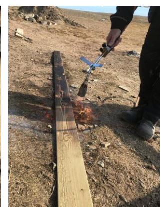
Left and middle: The rotten posts below the window. Right: The new wood is scorched with a gas burner to give it an authentic appearance.
