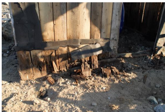
Restoration of Antonsens hytte [444] in Store Sødal. Top: The hut upon arrival. The bottom 15-30 cm of the walls were rotten. The boards in the corners and at the door were replaced to be able to carry the weight of the hut.
