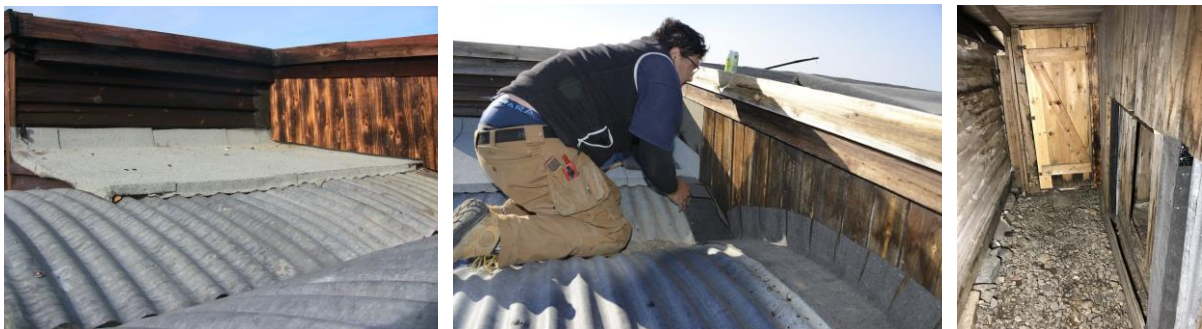
Left and middle: Roof over containers. Right: The hallway and opening into the containers.
