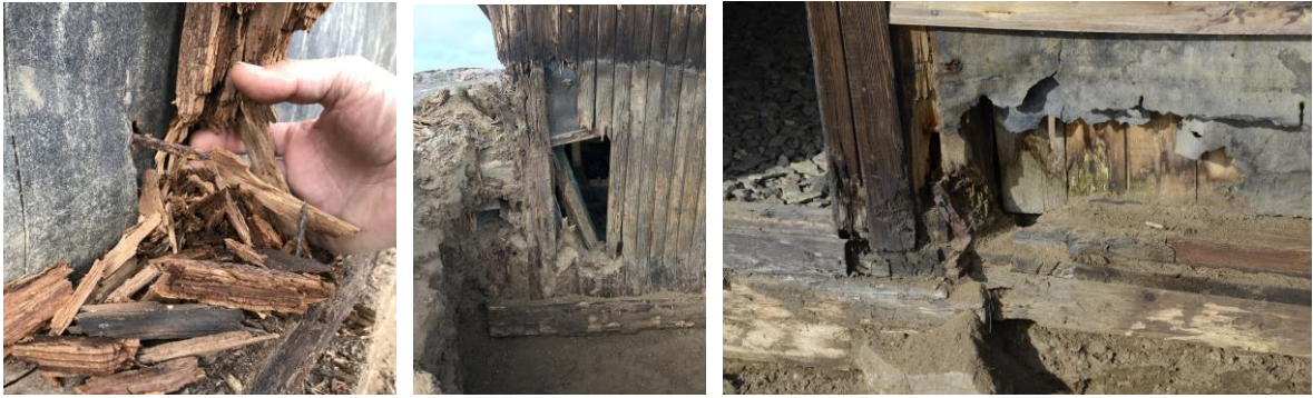
The excavation along the walls revealed more and more rotten wood, which practically disintegrated between our fingers.
