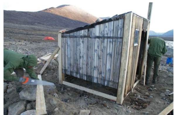
Restoration of Antonsens hytte [444] in Store Sødal. Top: The hut upon arrival. The bottom 15-30 cm of the walls were rotten. The boards in the corners and at the door were replaced to be able to carry the weight of the hut.
