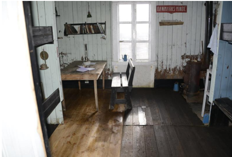
Left: Finished floor and skirting boards. Right: Drain from the floor is led through the bank.
