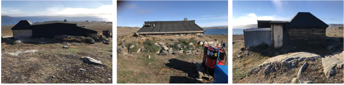
Villaen before restoration. Seen from North, West and East.
